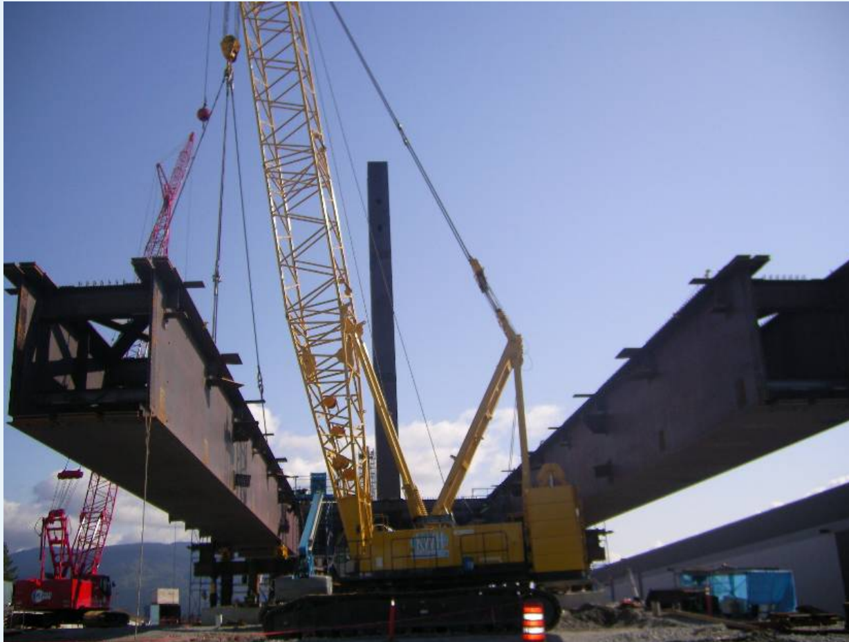
200-Ton crane squeezes between box girders
