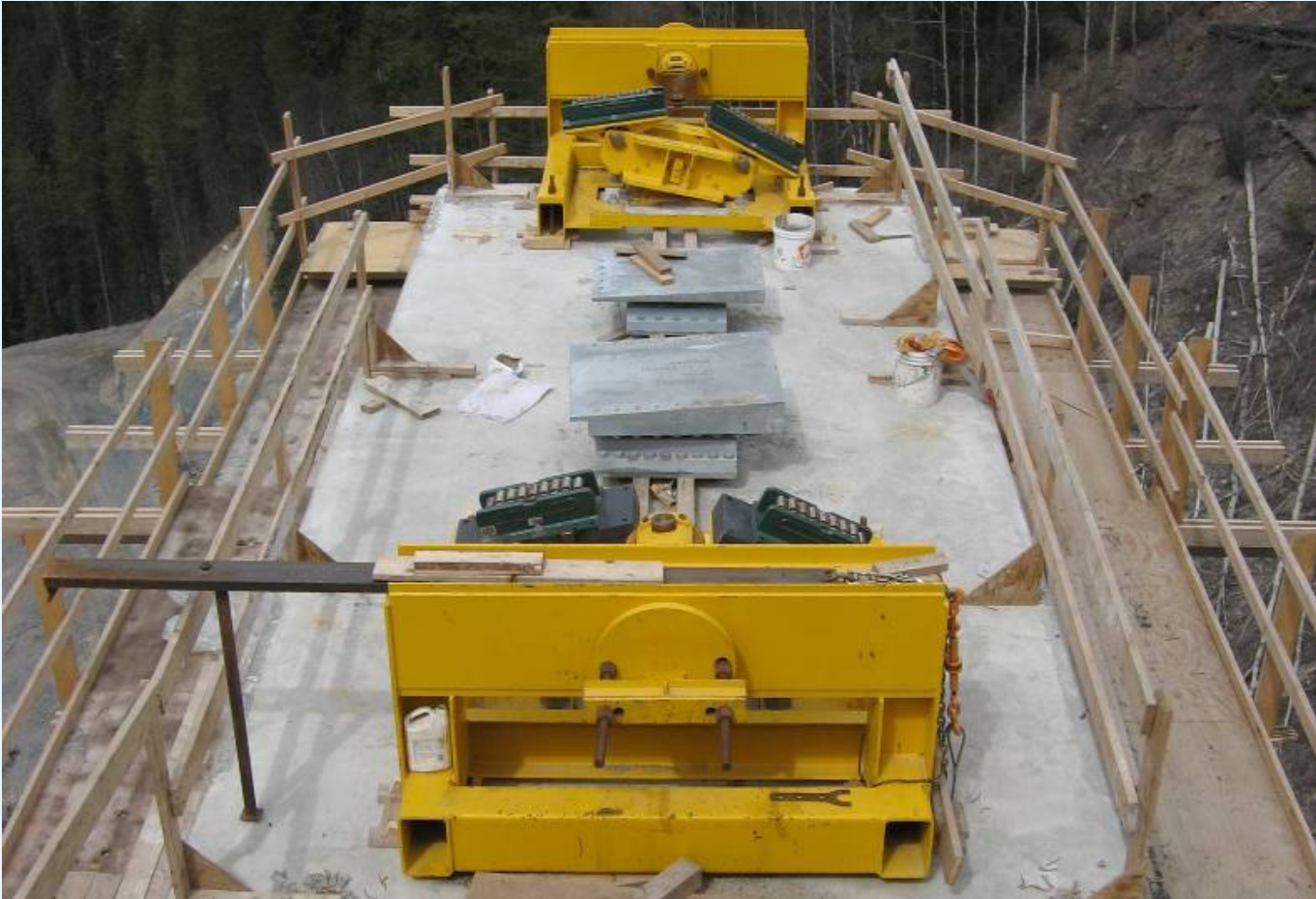
Note bearings preset on tops of piers for later installation
