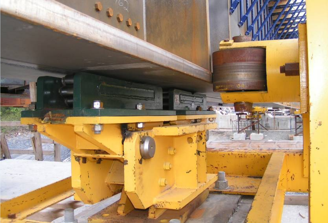
Close-up of rollers (green) and guide wheel
