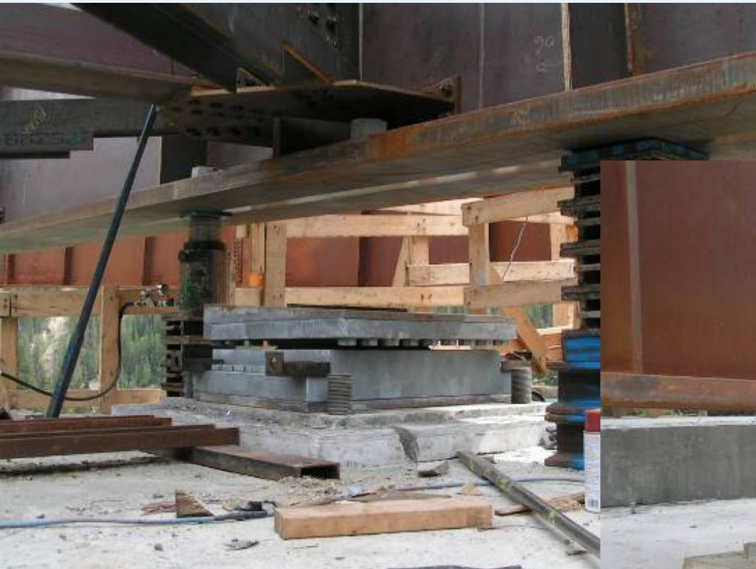
Bearing in position
