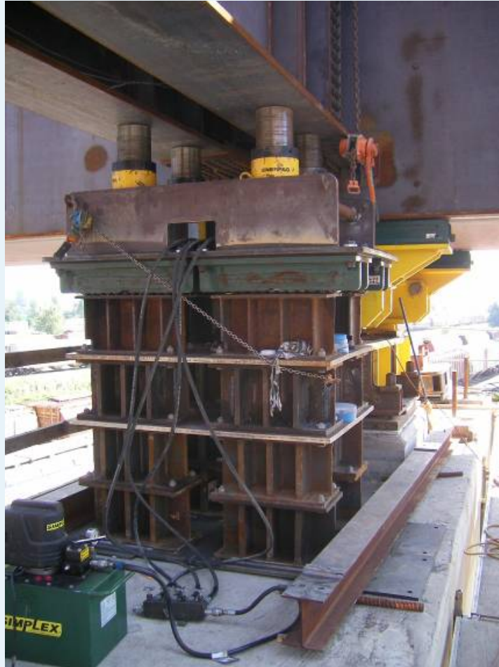
4-ft Jack Down with 700 tons load
