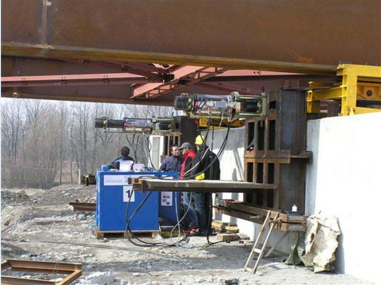
Launch system using two linked strand jacks pulling from abutment
