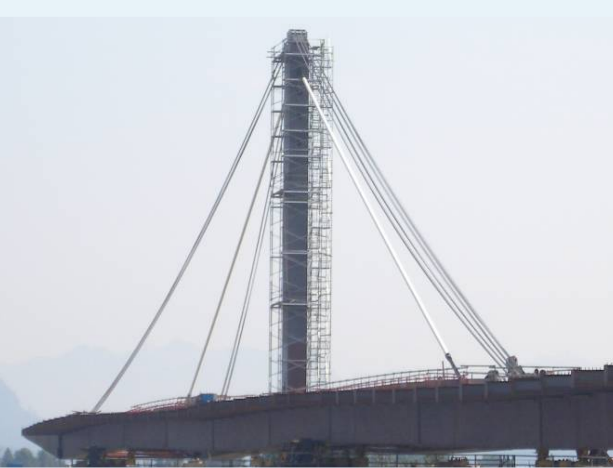
Used to lessen deflections for long launches
