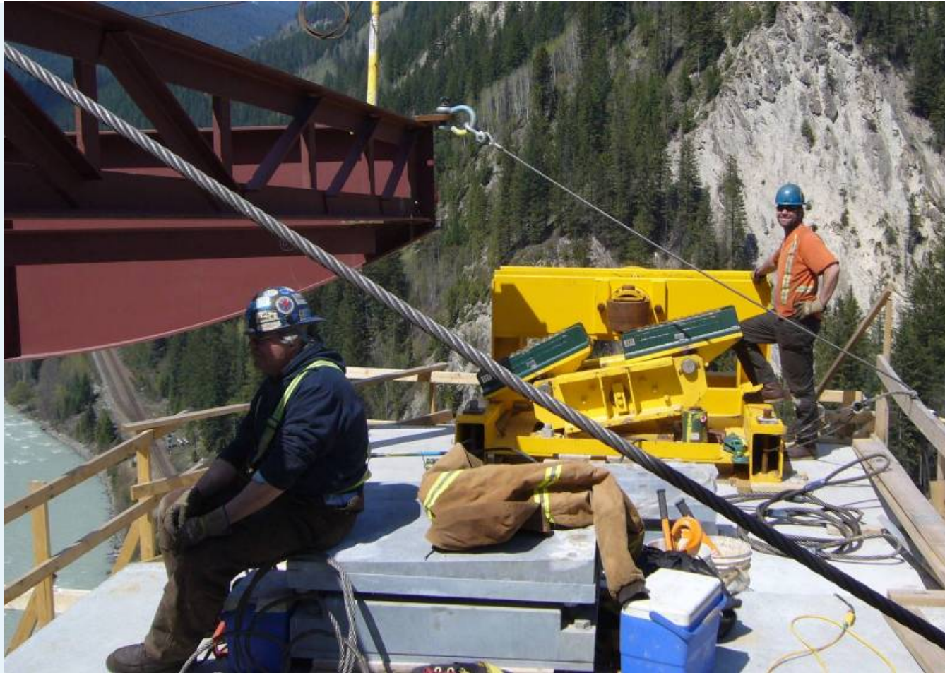
Nose about to touchdown on rollers
