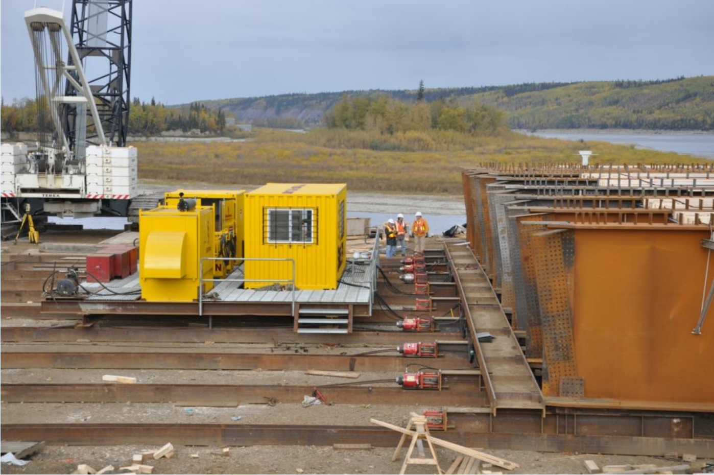
Using multiple linked strand jacks on steel rails behind abutment
