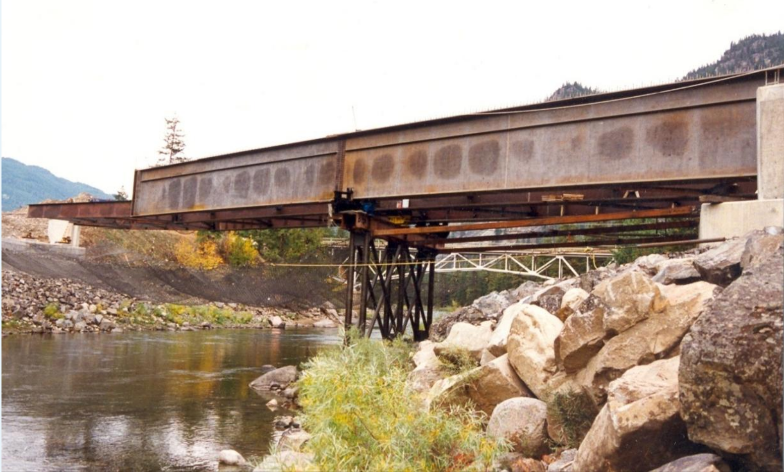
Simple temporary nose using rolled beams
