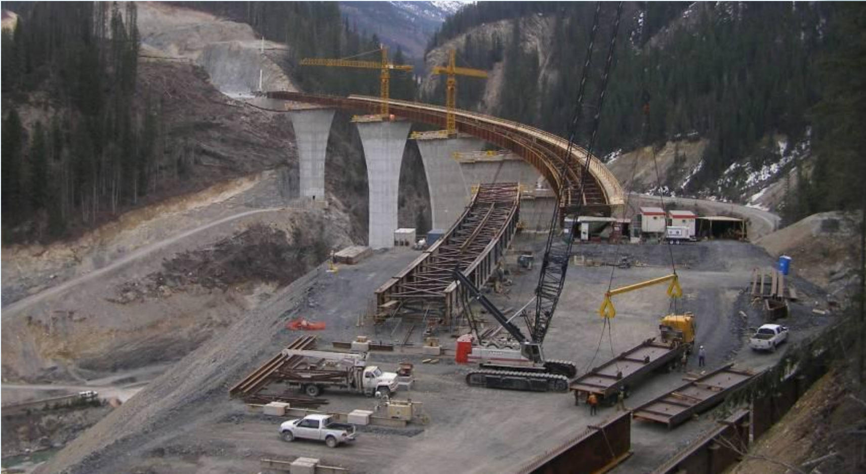
Girders assembled in "no-load" state, notice temporary supports
