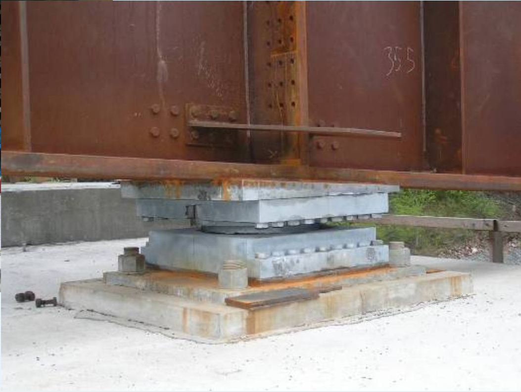
Bearing installed
